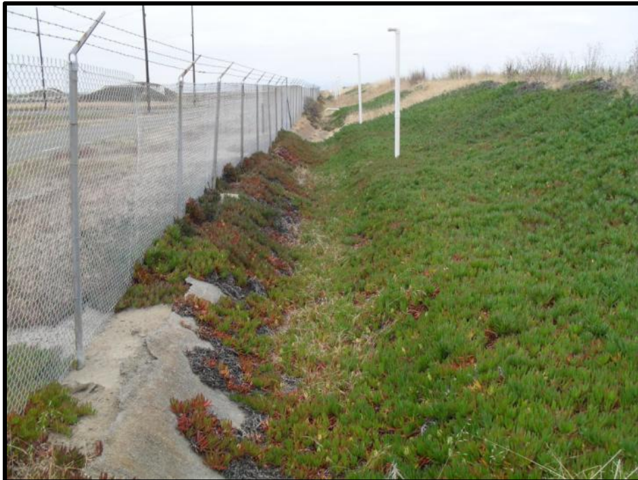
Concrete-lined drainage channel filled with ice plant, looking south
