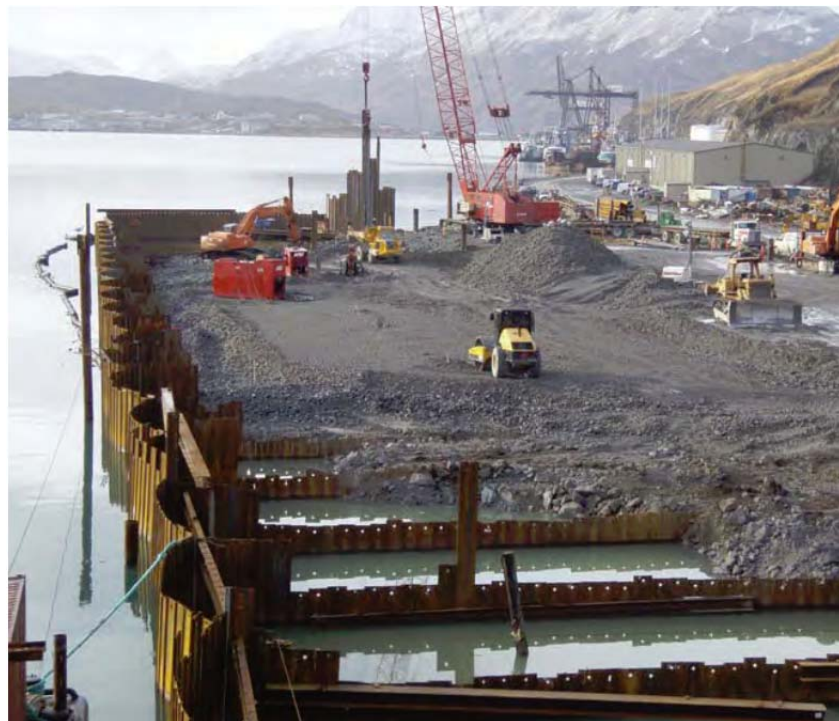
Figure 1. OCSPS during construction at Dutch Harbor Marine Terminal (OPEN CELL SHEET PILE Brochure 2010)
